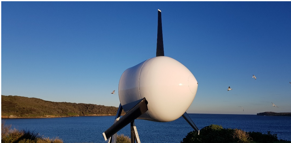
A MAKO.7 tidal turbine showing the unique patented bulb shape and the shorter blades which are possible with this design.
